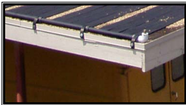
Collectors can be ordered in lengths that allow you to wrap your straps around the fascia.
