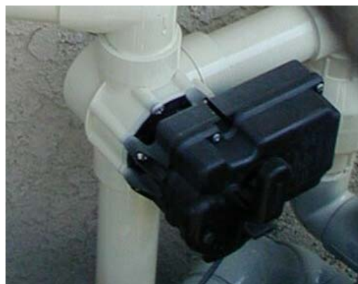
Compool solar valve and actuator.
