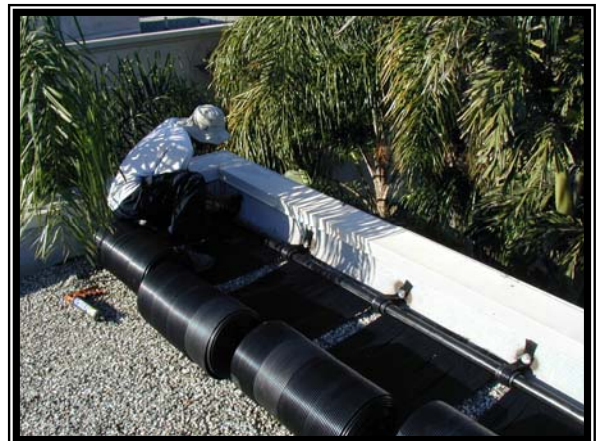
Straps can be made extra long so the bolts can go around the edge of a flat roof.
