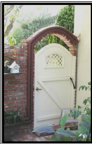
Flexible PVC was used to hide the pipes behind this brick archway.
