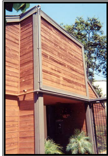
Matching paint can do wonders for camouflaging your pipe run.
