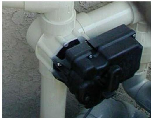
Compool solar valve and actuator.
